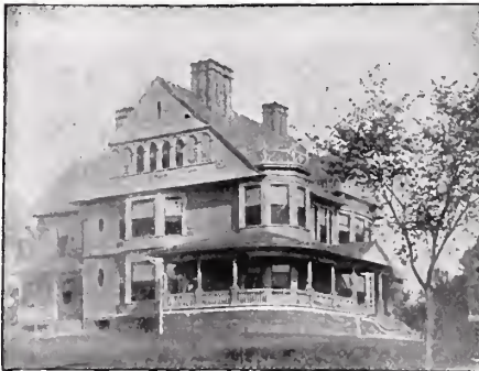
Residence of Frank M. Wilson, Willimantic, Conn. C. T. Beardsley, Jr., Bridgeport, Conn., Architect.
